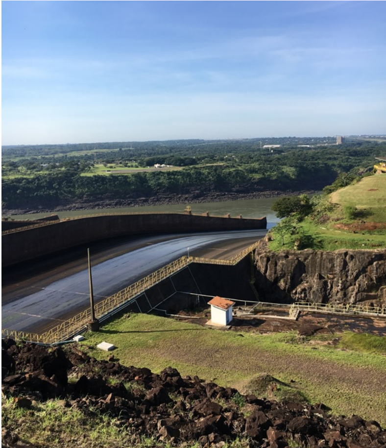
Figure 6.28. View of the spillway, view from the dam (without water).
