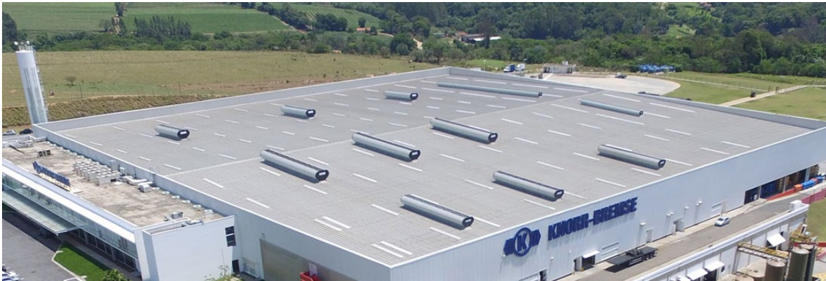
Figure 6.9. Real-life picture of skylights on the roof of the production building of the Knorr-Bremse plant in Itupeva, Brazil (2016).
