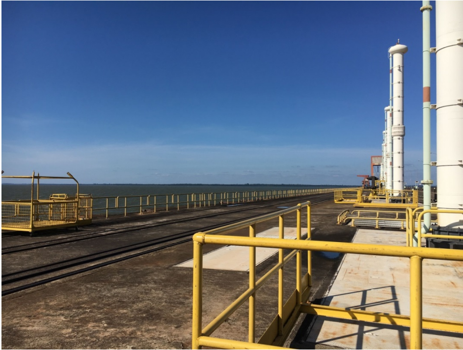
Figure 6.34. View from the dam on to hydrology element (Paraná River basin).
