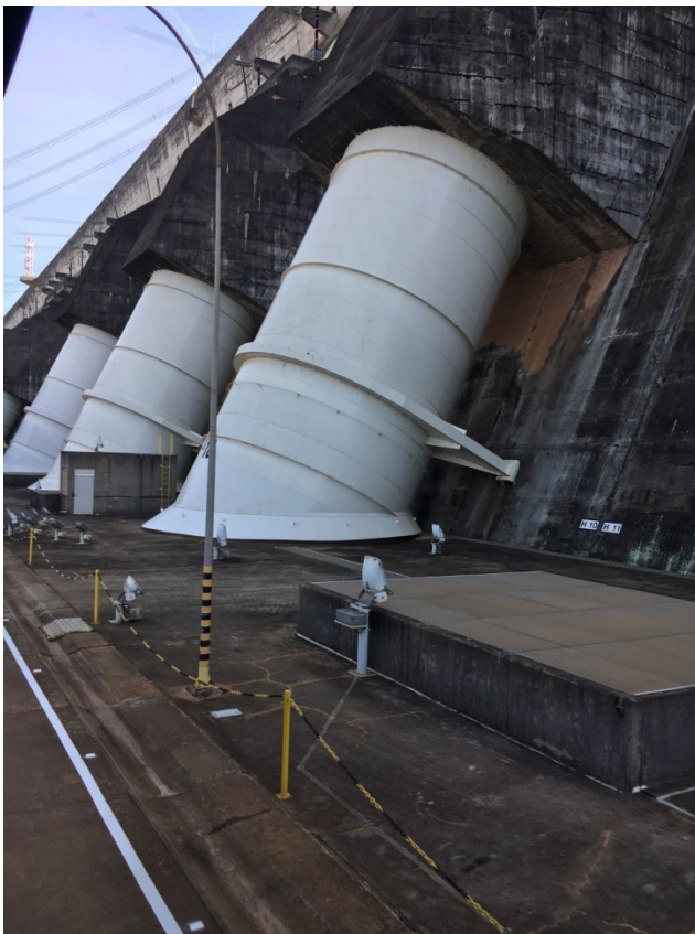
Figure 6.31. Tubes containing the generator units, close-up view.
