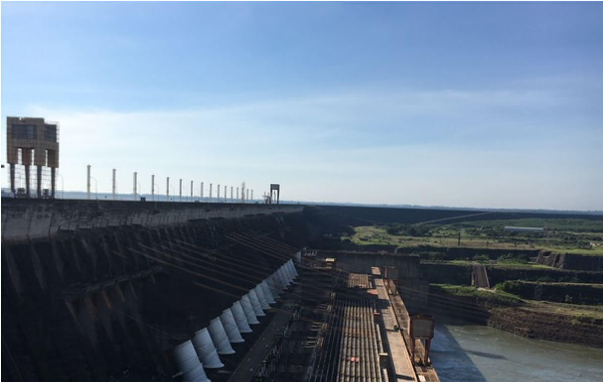
Figure 6.33. Concrete dam with road.
