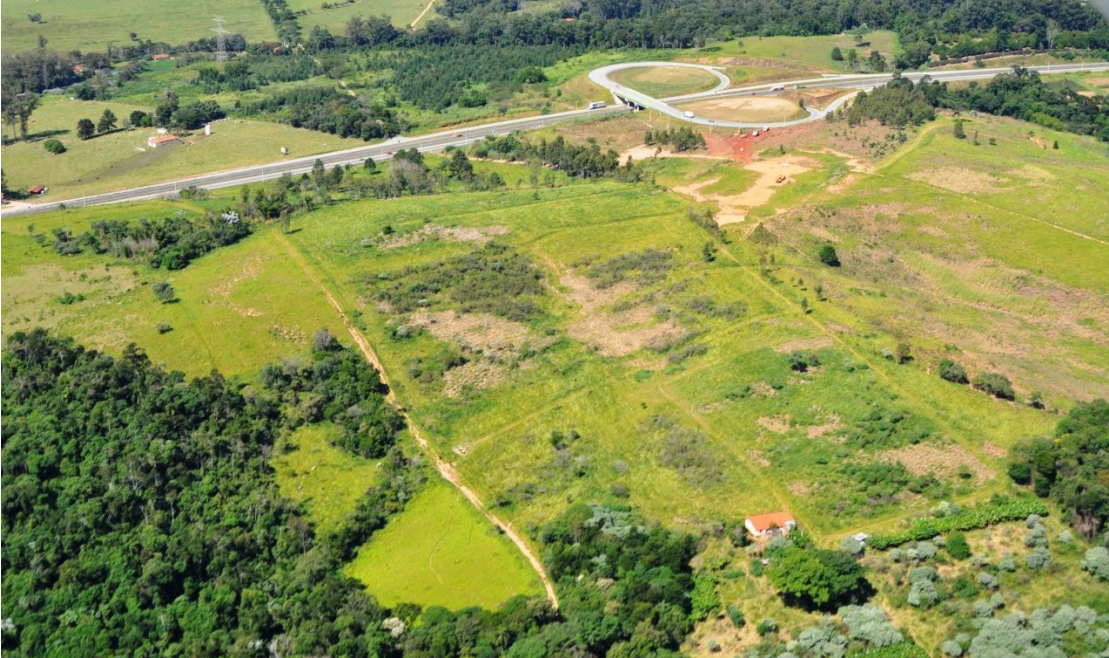
Figure 6.2. Land in May 2011, before start of construction.
