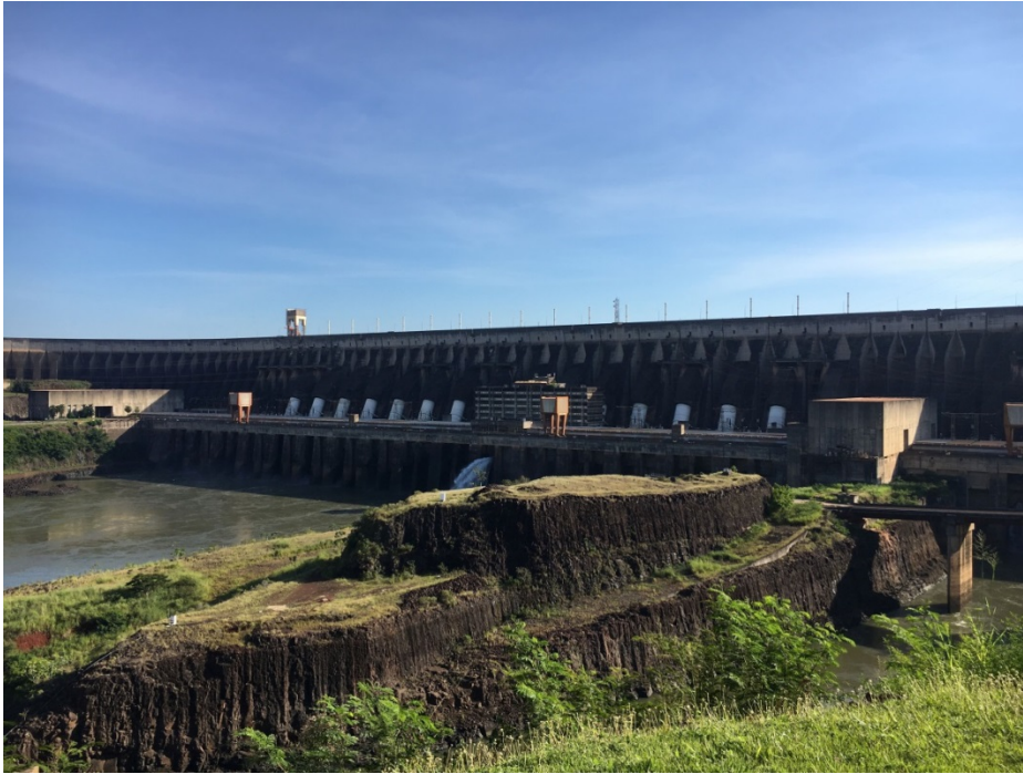
Figure 6.30. Tubes containing the generator units. Eleven out of 20 generator units are shown in the picture.
