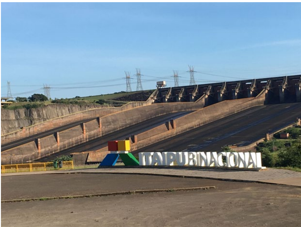
Figure 6.27. View of the spillway, front view (without water).
