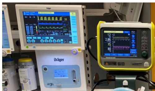
Figure 1: Ventilation devices in the operating theater.
